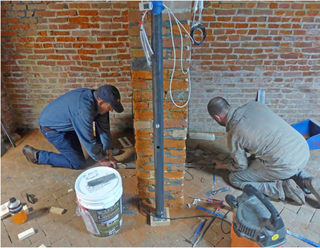
Image 9: Installing the damp proof course.
