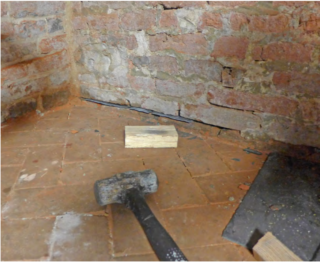
Image 10: Slate installed as a damp proof course.
